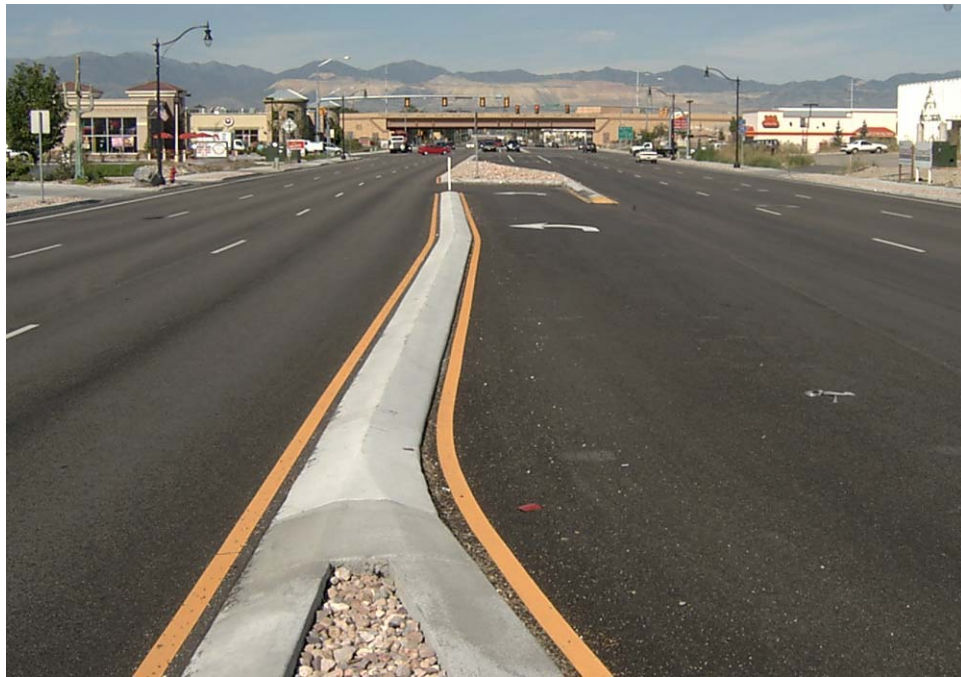
Figure 3-15. Raised median on 12300 South in Draper.
