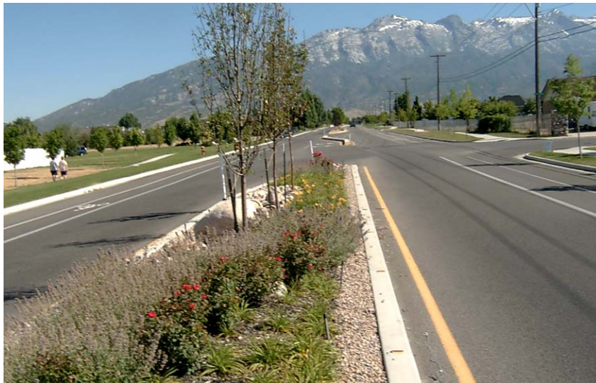
Figure 3-5. Raised median on SR 74 at 10000 North.
