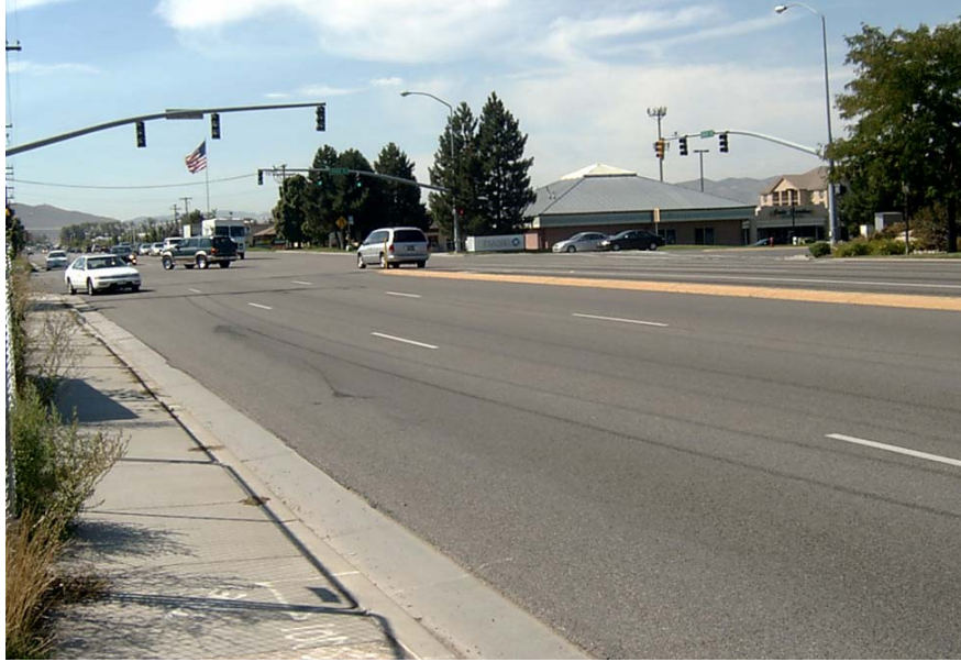
Figure 3-7. Raised median on State Street at 10600 South intersection.
