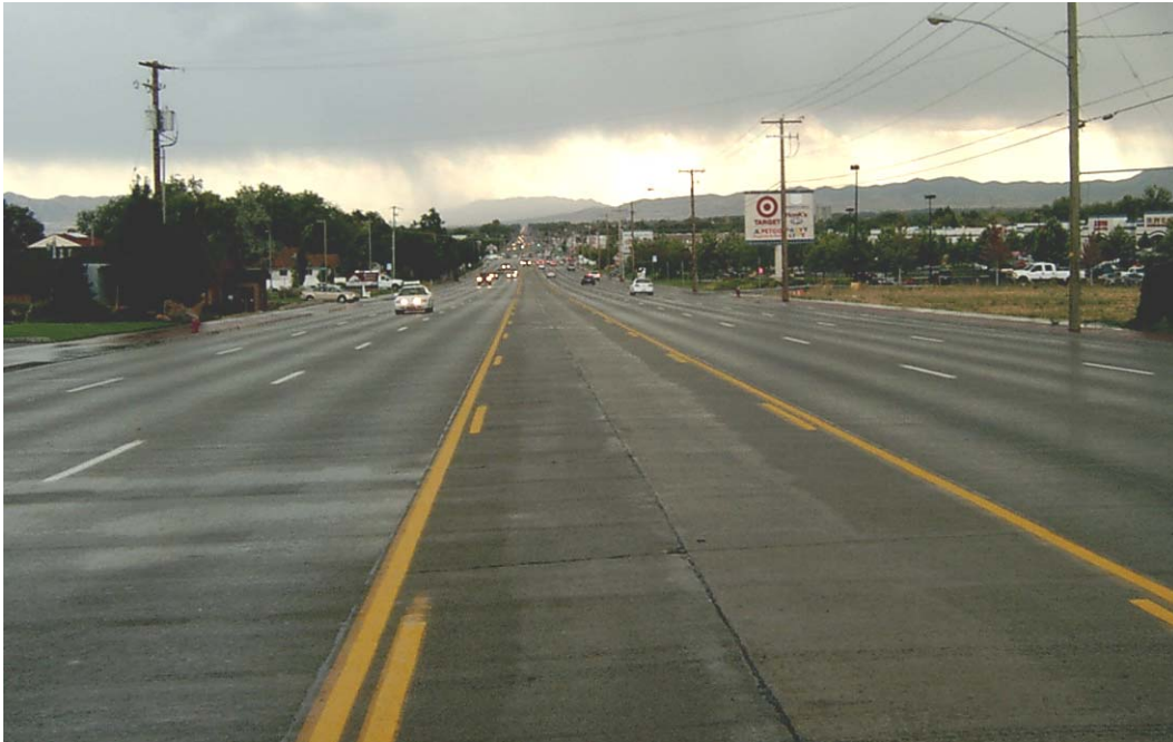
Figure 3-16. TWLTL on Redwood Road near 7000 South.
