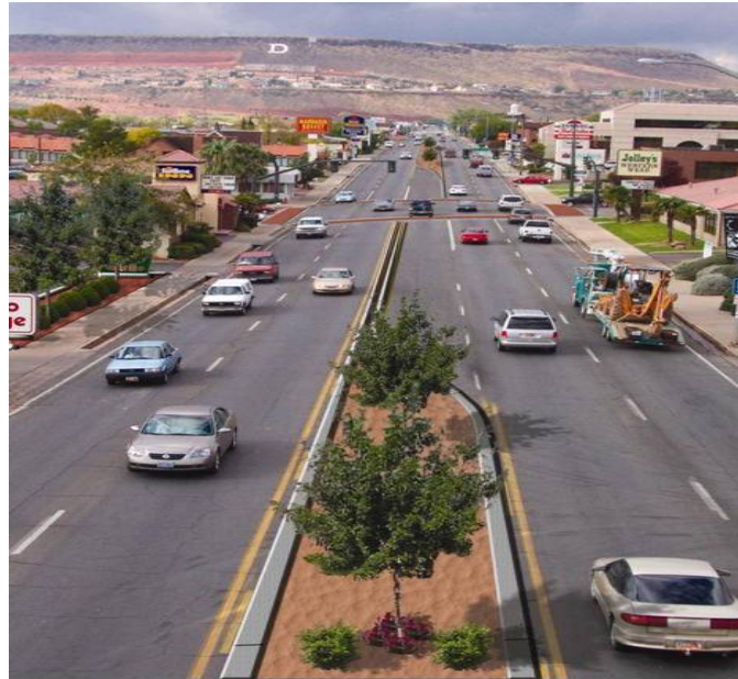
Figure 3-17. Artistic rendition of the future raised median on St. George Blvd. (UDOT 2005a).
