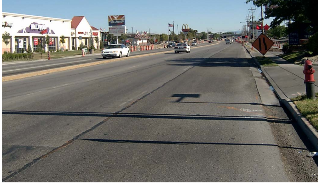
Figure 3-10. Raised median on Redwood Road near 5400 South.
