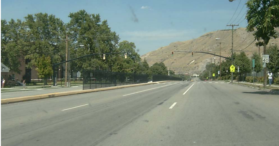
Figure 3-9. Raised median on 300 West near West High School at 200 North.
